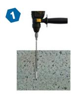
1. Using a carbide-tipped drill bit complying with ANSI B212.15-119, drill the hole 1/4 inch (6.4mm) deeper than anchor embedment.
